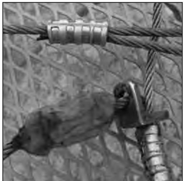
Applied Nycopress clamp covered with silicon glue
